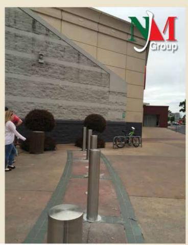
This installation at Epping Plaza features fixed sub-surfaced mounted bollards. The base plate gives it a nice professional aesthetic.
