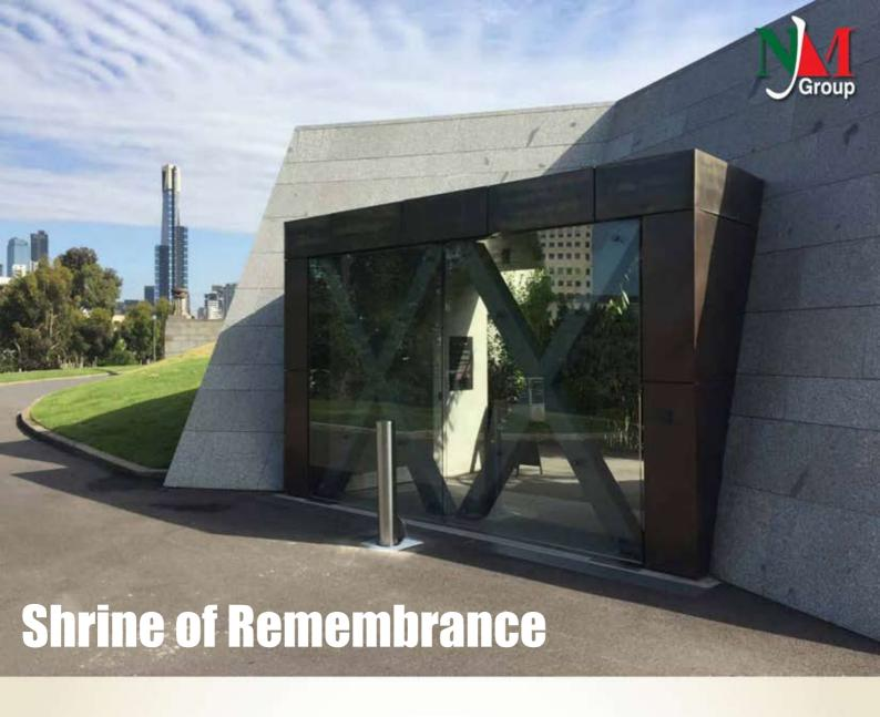
This installation on one of Melbourne most iconic buildings features stainless steel bollards. The bollards are removal which means if necessary it can be taken out and then returned and locked into place with a key. The bollards are sub-surfaced mounted which means the base of the bollard is installed below ground.
